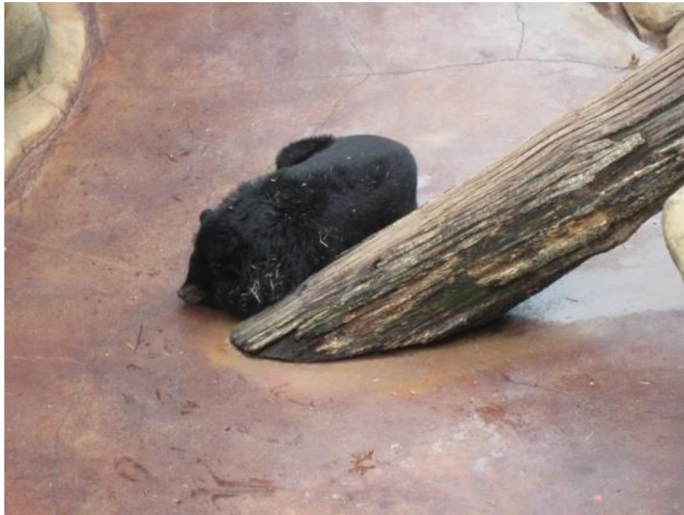
Cracks in cement floor in bear pit at Three Bears (Feb. 4, 5, 2014)
