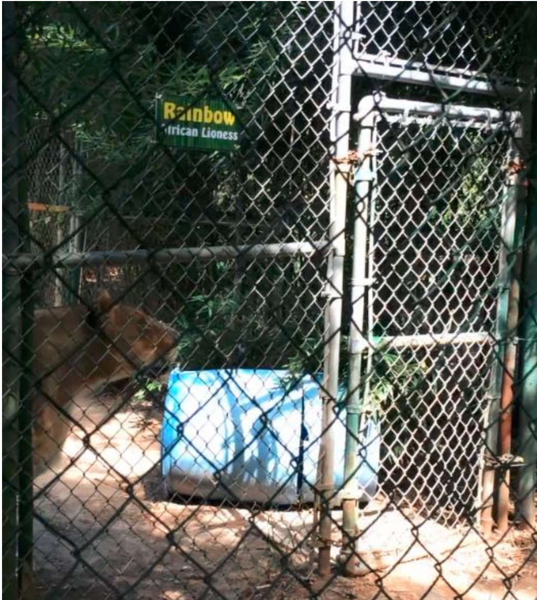
Photo 14: The frame of the gate to the lion enclosure is rusted (7/29/14)
